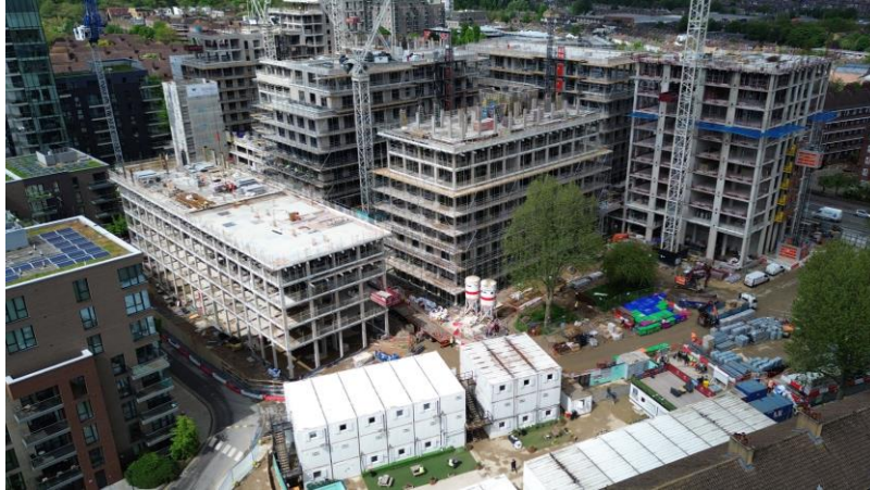
Concrete superstructure developing
