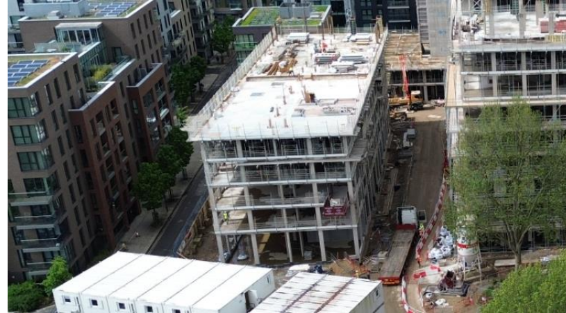
Concrete frame advancing on B4 & B5
